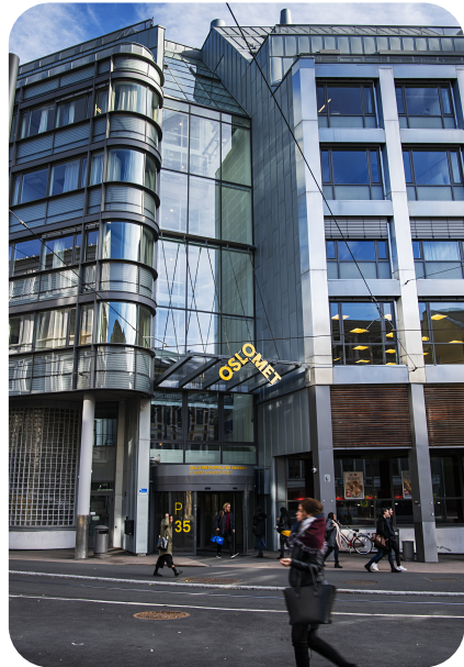
Figure 2.1: View of the entrance to P35 from Holbergs plass.
